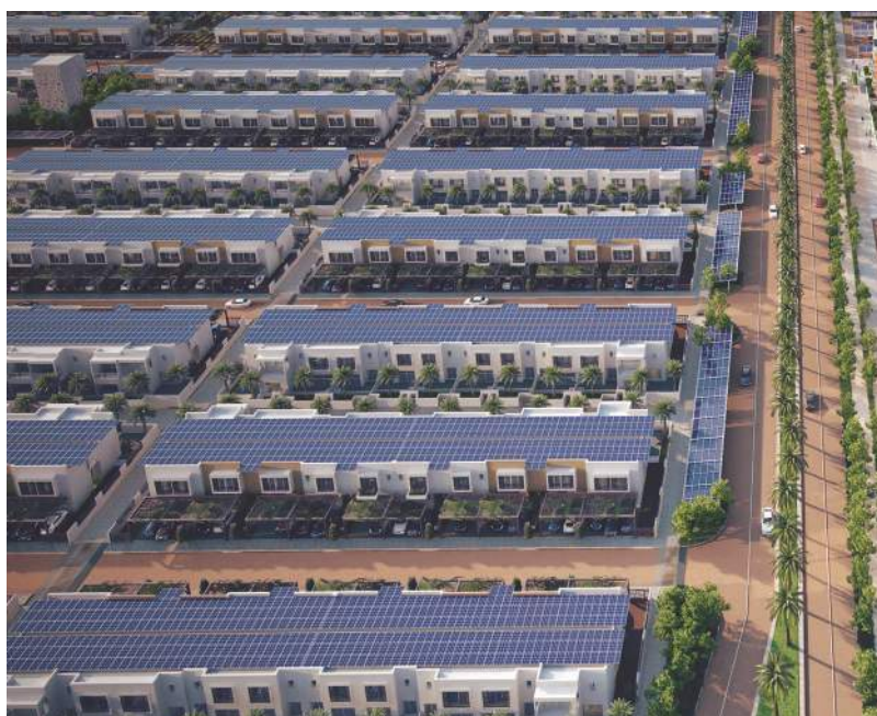
Solar panels are being used in new developments in Sharjah to generate electricity and treat wastewater
